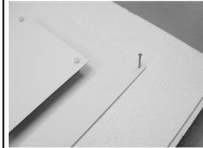
**2.** Insert 2" long screws from toggle bolt through each corner hole on back plane of CX-22 (4 places). Push through ceiling tile material.
