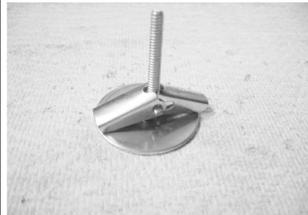
**3.** On back side of tile, place large washer over screw end, flat against ceiling tile and screw toggle wing into place as shown. Repeat for each corner.
